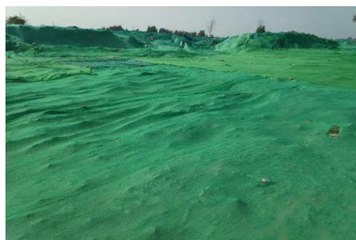
Covering exposed loess on site
